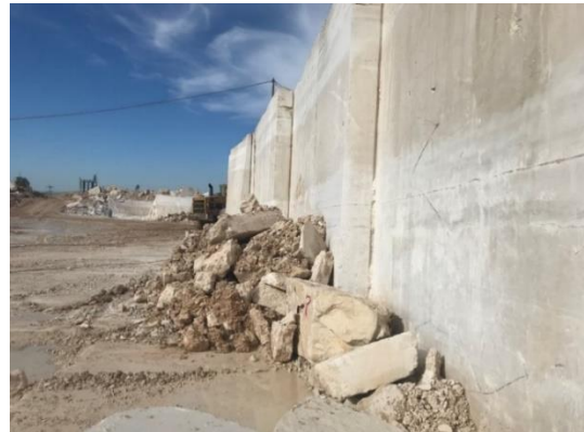
Fig. 3. An under working bench face of the mine.
