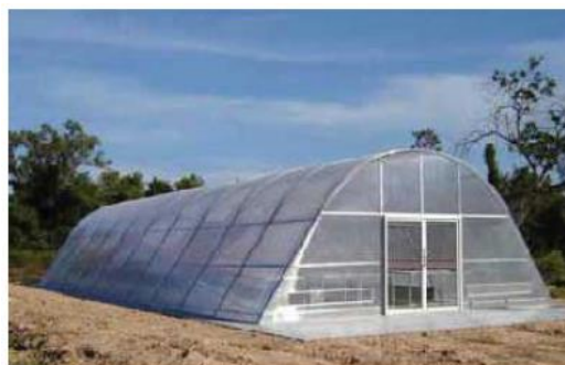
Figure 5: Pictorial view of greenhouse solar dryer used for chilli drying in Thailand [32]
