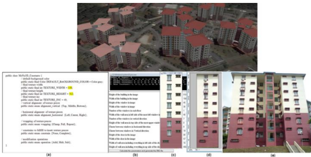
Figure 10. The process of generating the façade via DPF and visualization in Google Earth was accepted by the Google Earth 3D community. (c) is the procedurally generated texture (15KB). (Kolej Perdana U4B, UTM, Johore Bahru, Skudai, Malaysia)
