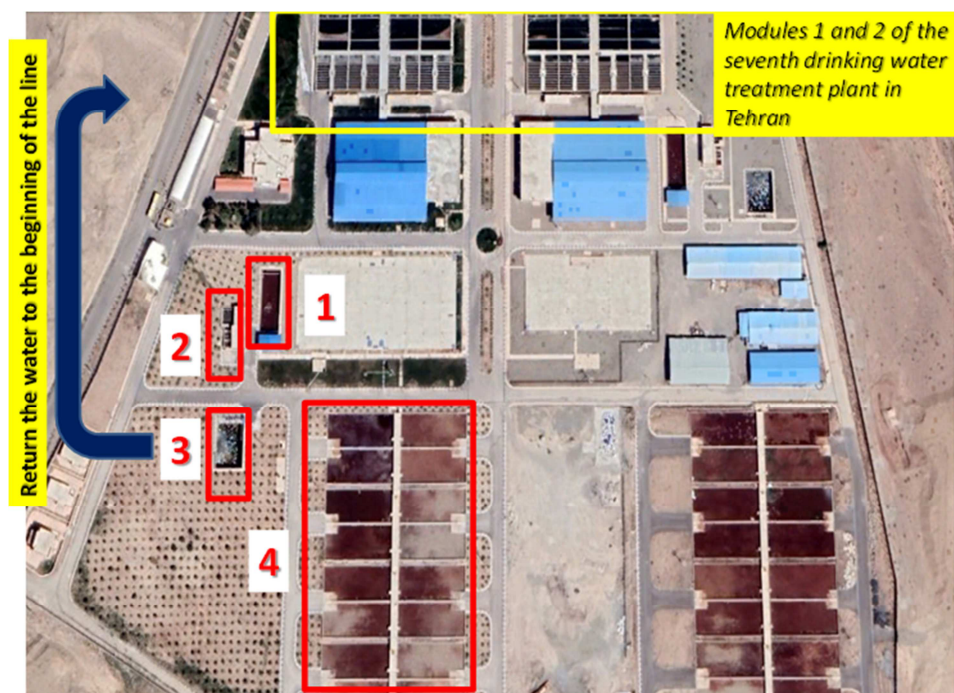
Figure 7. Aerial image of the seventh Tehran water treatment plant
