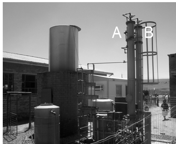
Fig. 1. The biofilter system analyzed in this study. Label A indicates the iron filter, label B the manganese filter
