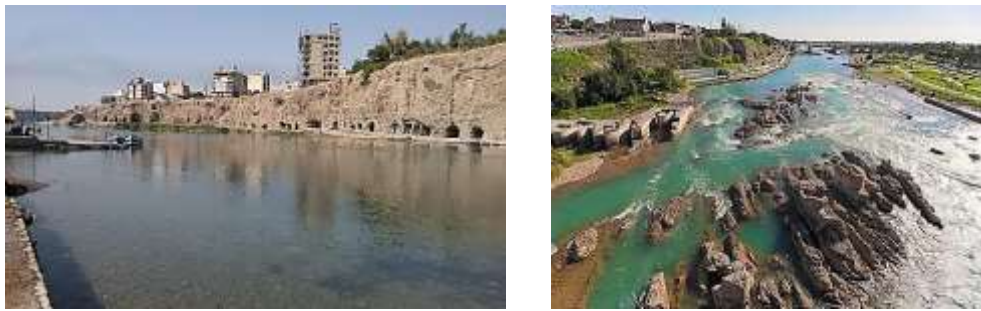
Fig 3. General View of river
