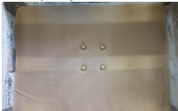
c) Step 2. Driving the piles in sandy layer
