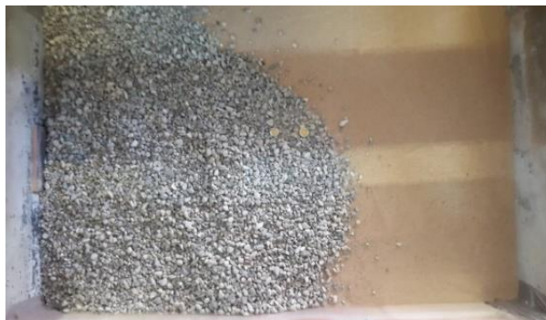
e) Step 3. Filling the gravel (10 cm)
