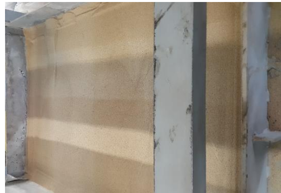
b) Step 1. Filing the box with sand (90 cm)
