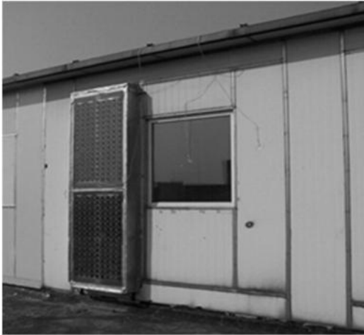
Figure 1. Photovoltaic Trombe wall
