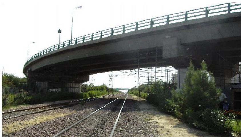
Fig. 2. Access railroad between piers 3 and 4
