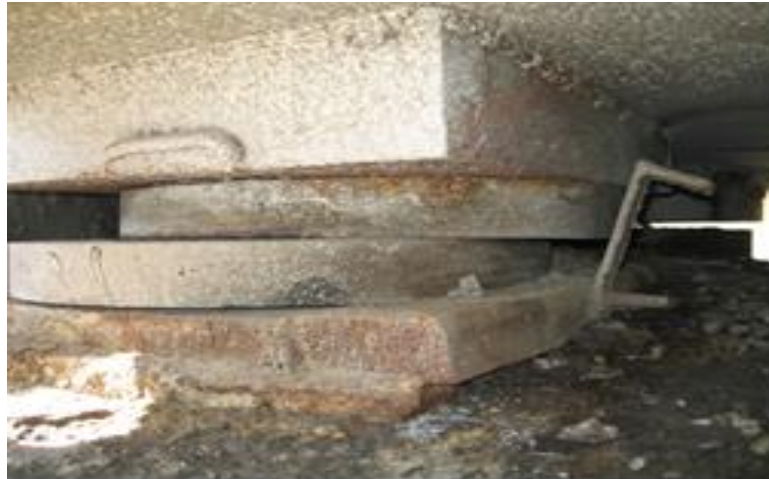
Fig. 20. Elastomeric bearing of lateral movement in the Ghale Morghi bridge
