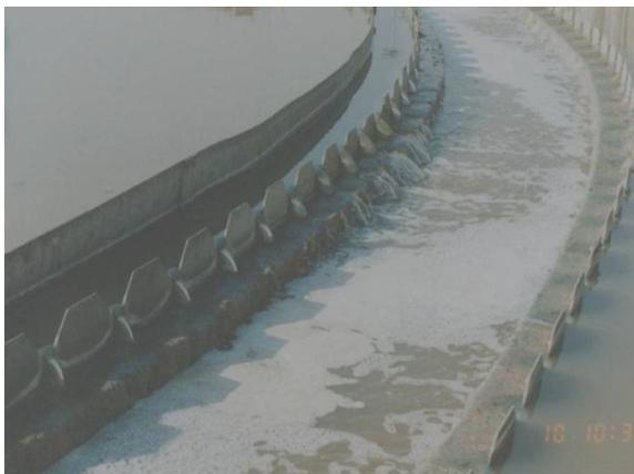
Fig. 3. Sample of unsuitable construction work (unbalanced V-notch) (Amir AIMOUR, 2008).
