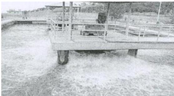
**Fig. 9.** Surface aerators cause lower BOD removal efficiency.
