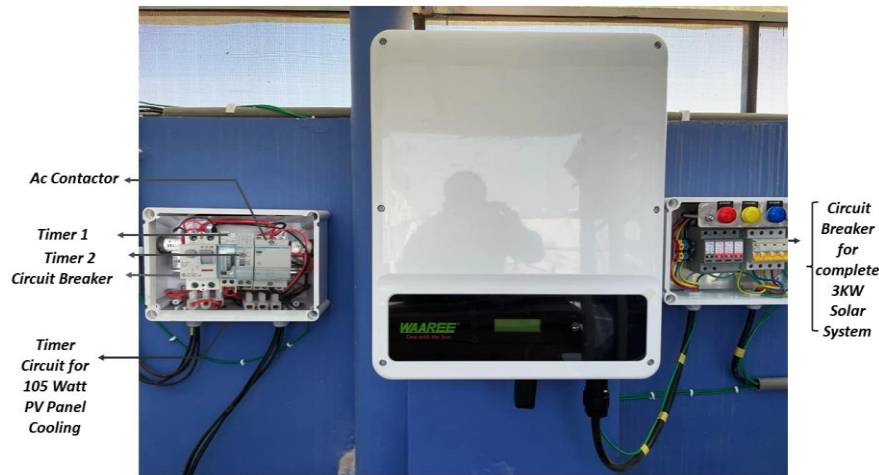
Figure 13. The connection actual layout for cooling the Photovoltaic Panel on the timer
