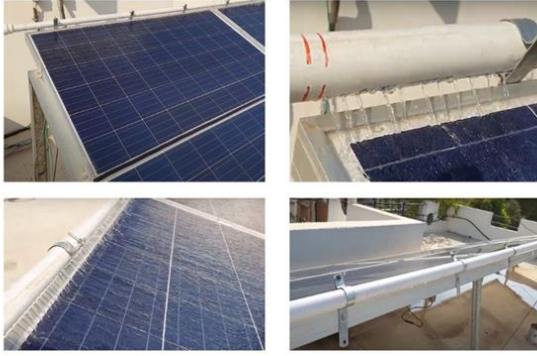
Figure 6. The configuration of the PV system includes movable 105-Watt Solar panels and a spray system for cooling the PV panels from various perspectives
